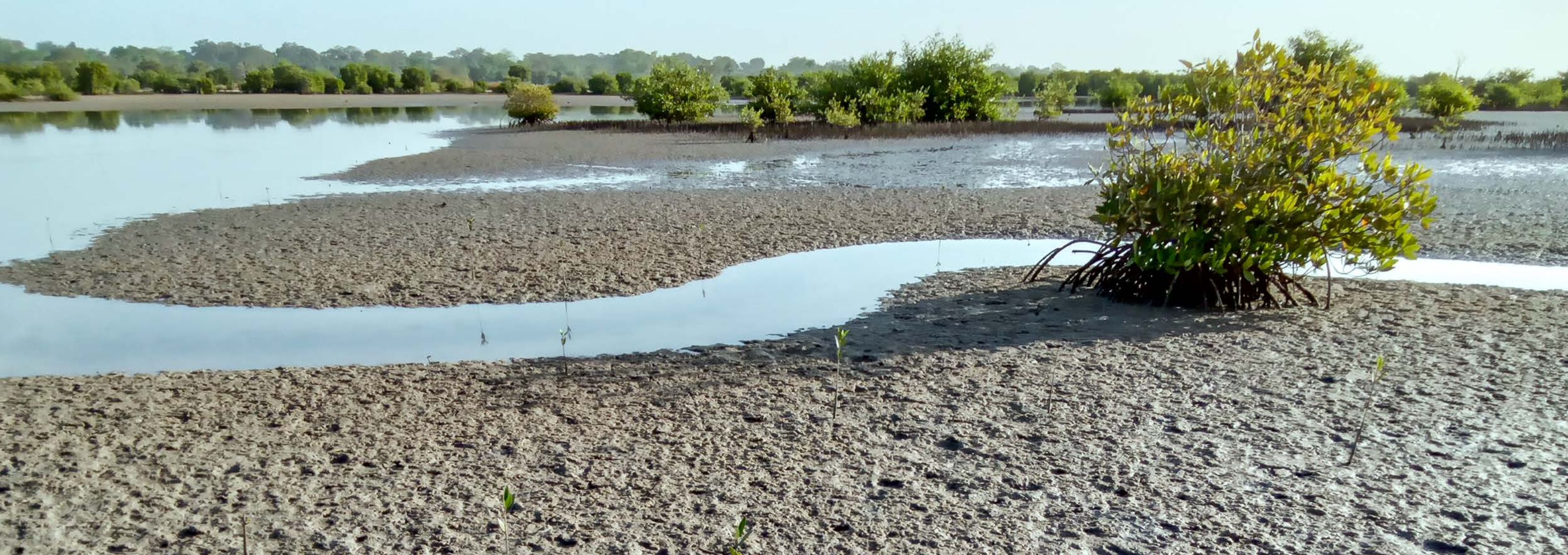
Channel for hydrological restoration to enable natural mangrove regrowth.
