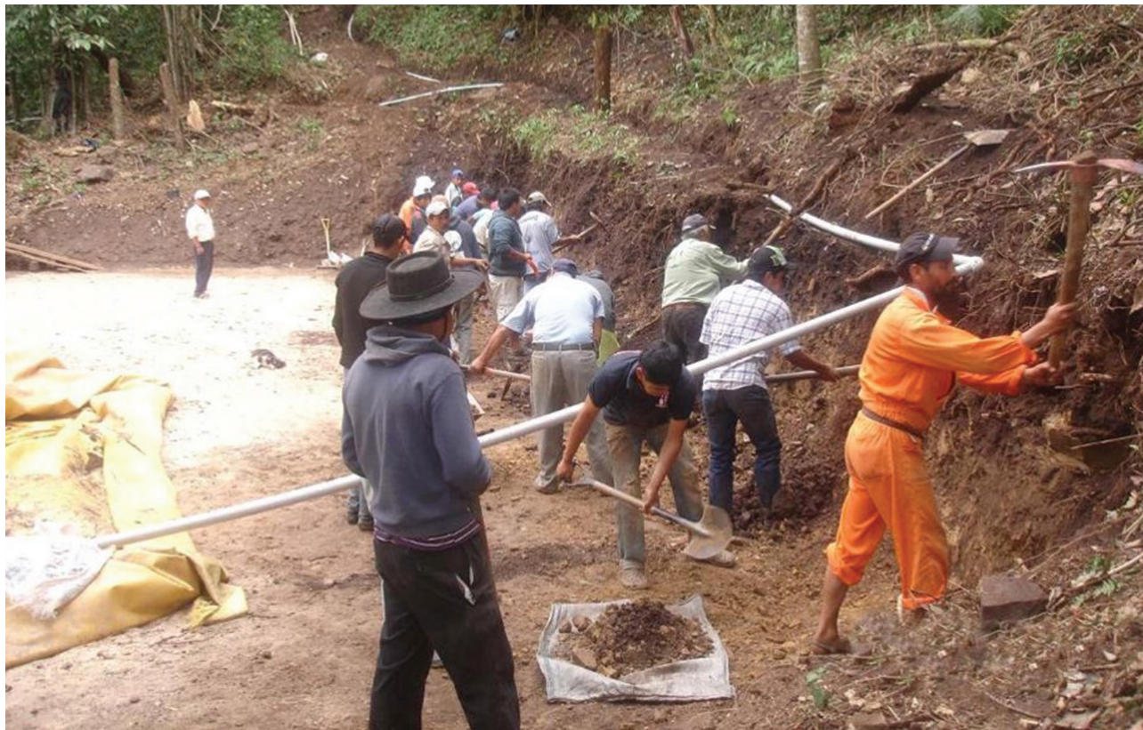
Excavation work by the community members for the water tank installation
