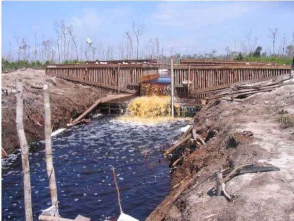
Dams constructed to prevent further drainage, Central Kalimantan.
