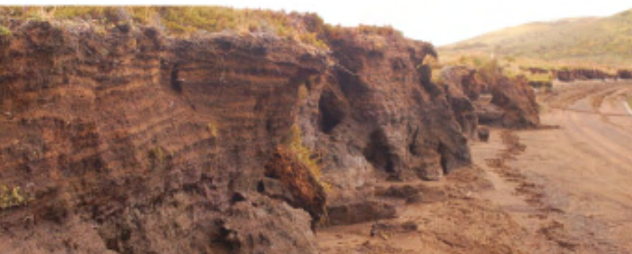
Sea level rise may lead to erosion of peatlands by wave action (Tierra del Fuego, Argentina)
