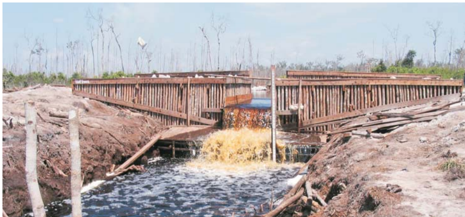
Sebangau SPI channel, dam constructed to prevent further
