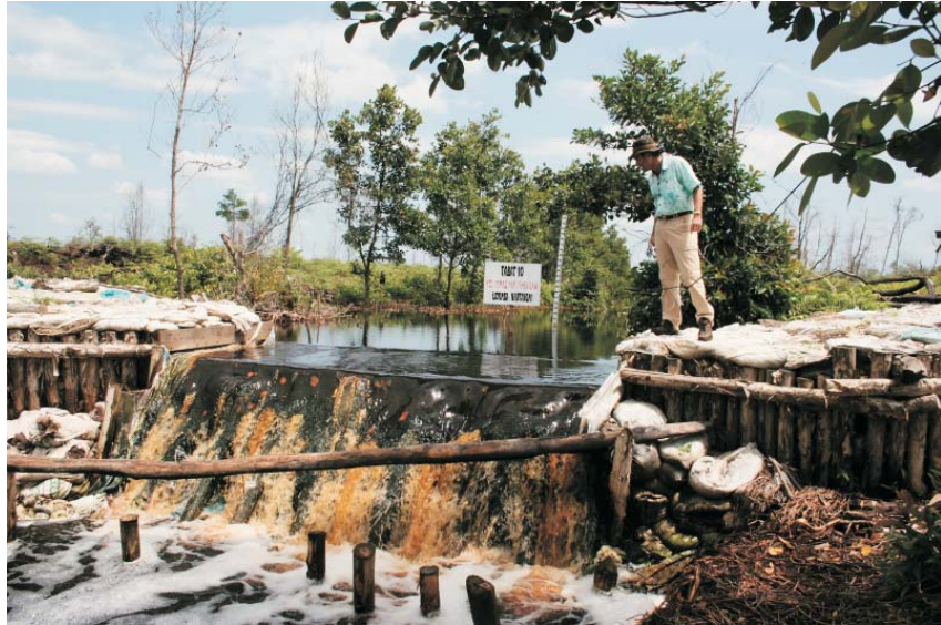
CKPP dam no. 10 in block A north
