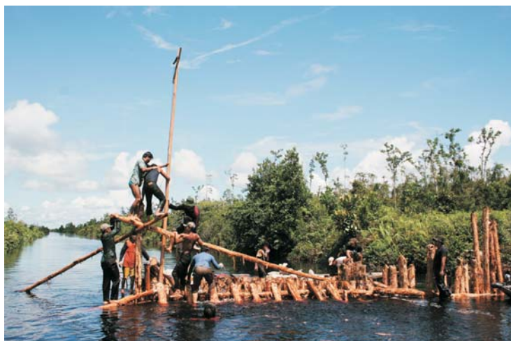
Community involvement in peatland restoration -blocking drainage channel
