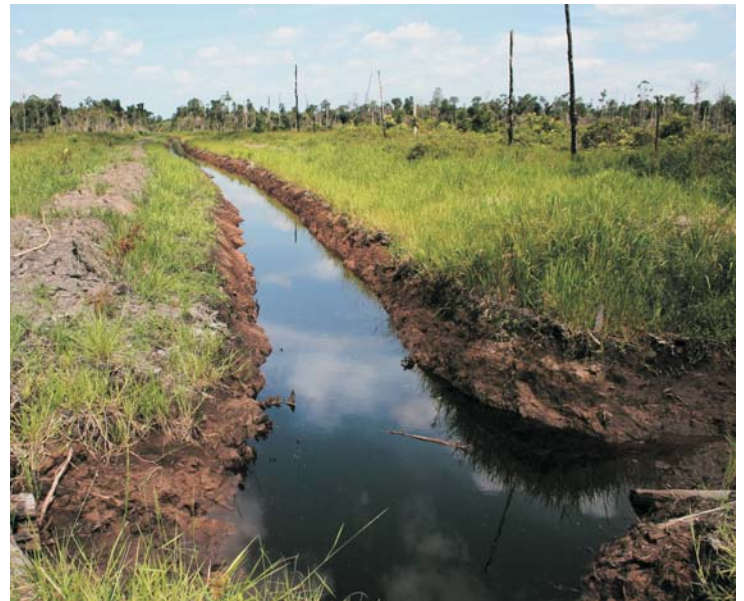
New drainage channel in Block A in shallow peat
