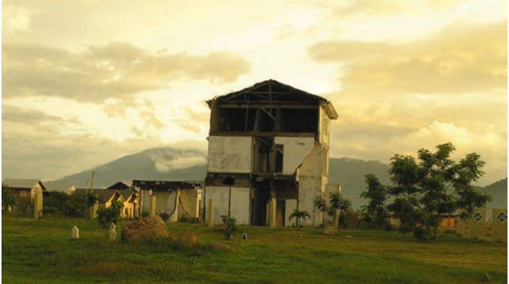
Tsunami damage in Banda Aceh, Sumatra. Photo: Pieter van Eijk.
