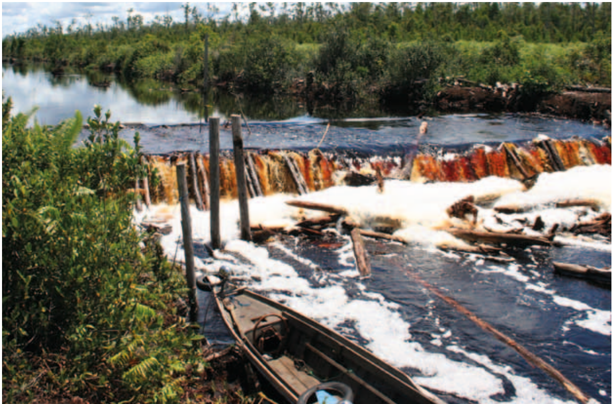
Our advocacy at the UN Climate Talks and Copenhagen Conference is based on our research and field experiences in peatland management; this is a dam in Hell's Canal, Central Kalimantan, Indonesia built to increase the water level leading to vegetation regeneration. By Marcel Silvius.
