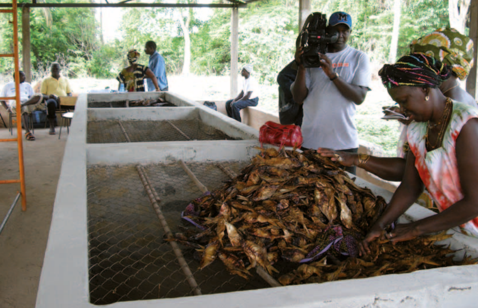
These newly installed fish smoking ovens in Canaméne, Guinea Bissau use six times less fire wood per kilogram of smoked fish, thereby significantly reducing the impact of this activity on mangroves, from which the firewood is collected. By Richard DaCosta.
