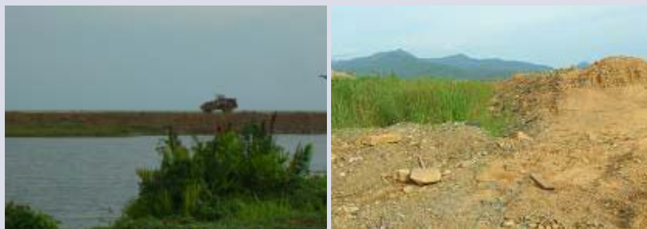
Figure 66. Swamp defragmented by highway construction
