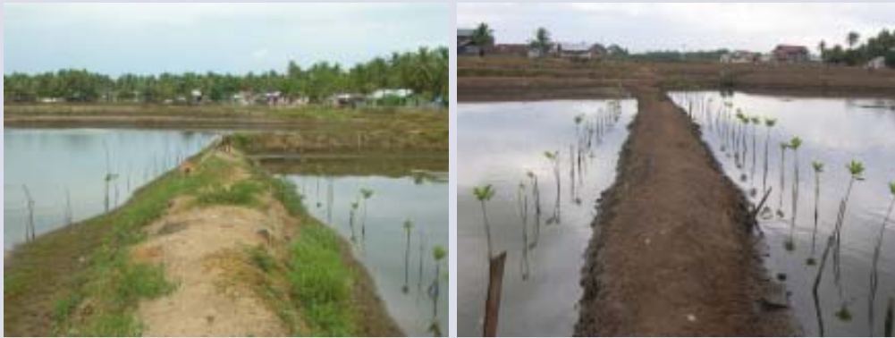
Figure 57. Left: Gently sloping embankment (prone to attack from livestock), Right : Steep sided embankment (relatively safe from attack by livestock)
