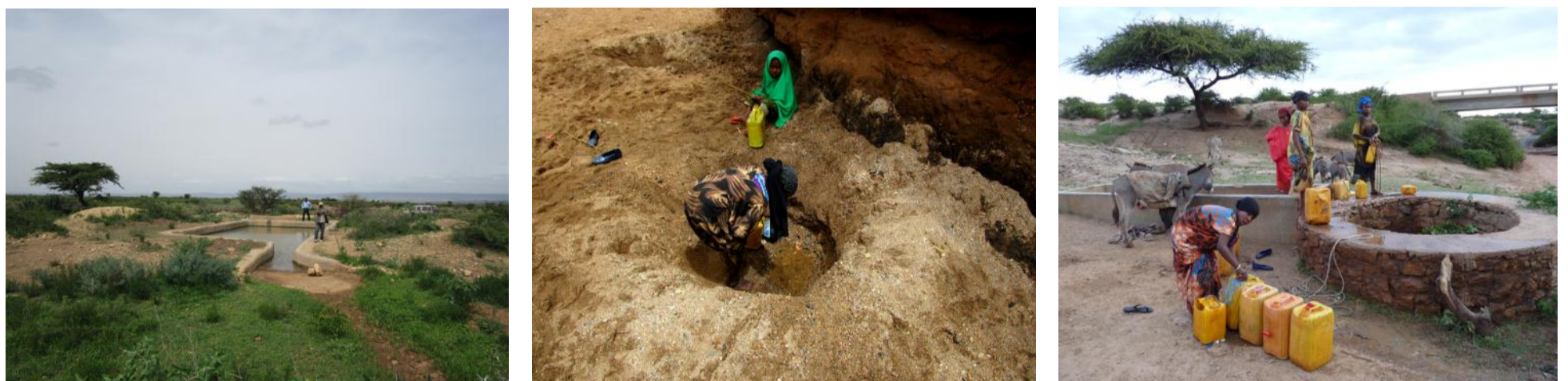
Figure 4.2 Different types of water sources present in the project area. From left to right: birkad, scoop hole and lined shallow well.
