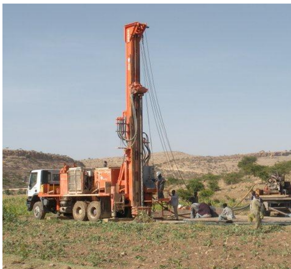
Figure 4.8 Borehole drilling in Ethiopia (www.dando.co.uk, 2016).
