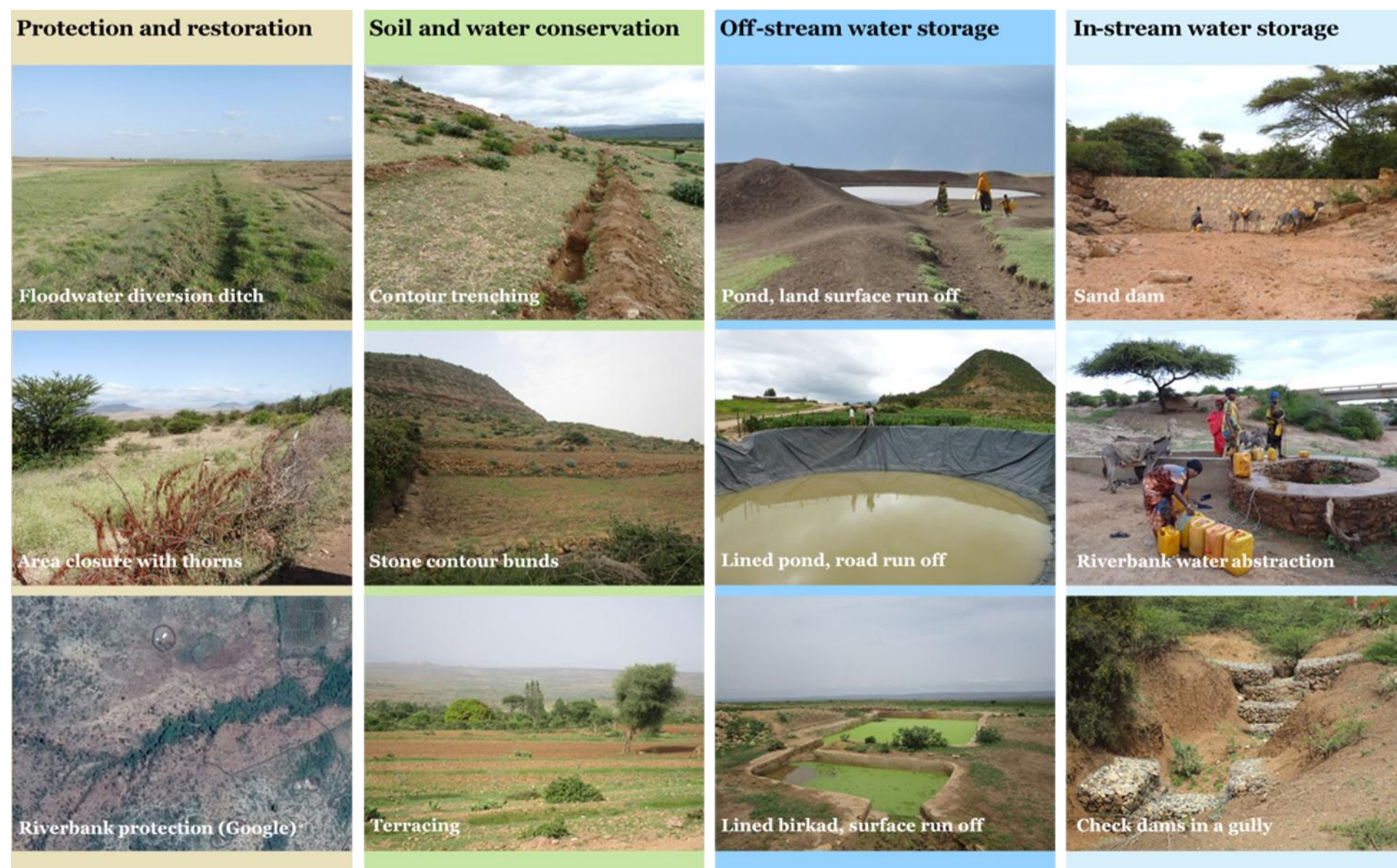
Figure 5.1 Examples of ecosystem restoration interventions. All pictures taken by Acacia Water in the project area. Strengthening ecosystem services is essential towards building resilience. Landscape characteristics dictate which ecosystem restoration interventions are most suitable for a certain location.
