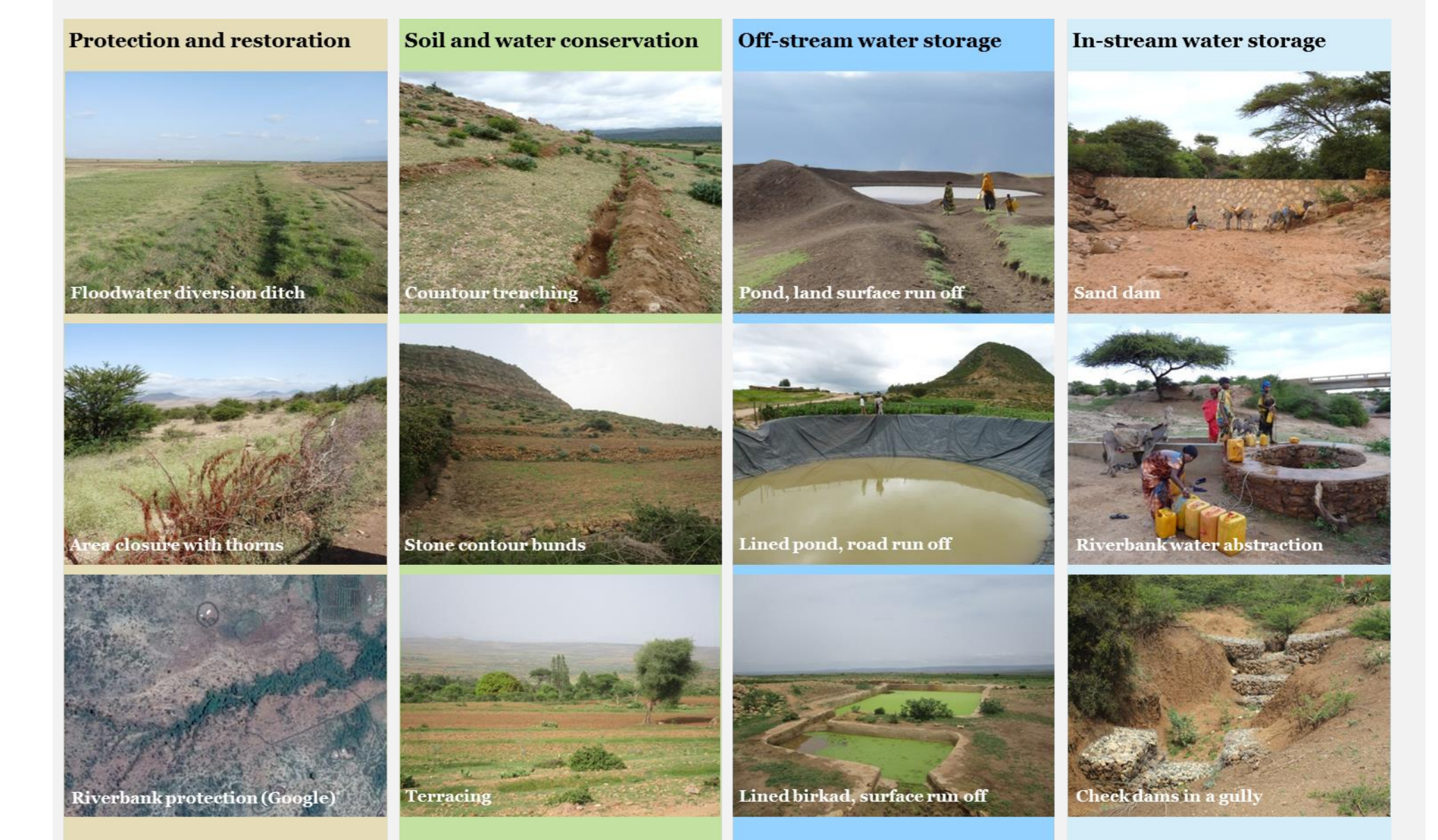
Figure 1. Examples of ecosystem restoration interventions organized per type. All pictures taken in the SCRSE project area by Acacia Water.
