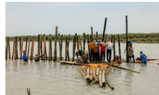
Figure 21. Placement of vertical poles and other components © Deinar Santayana, Witteveen+Bos
