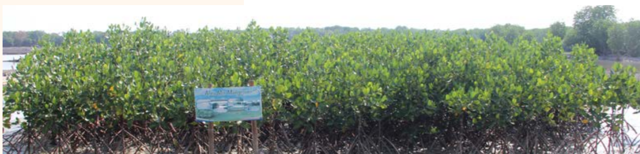
Figure 6d: AMA 6 months after construction in Tambakbulusan (© Suhadi, Blue Forests)
