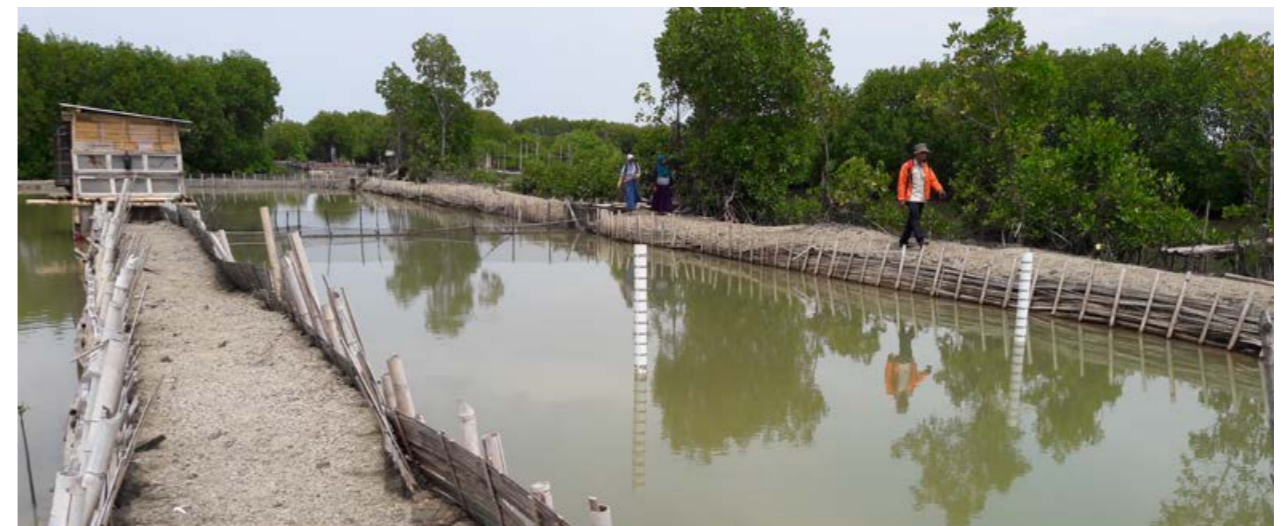
Figure 12: An image of the new dyke with the bamboo screens, attached to each other with iron wire, still in place, and the old river dyke in the background (© Roel Bosma)
